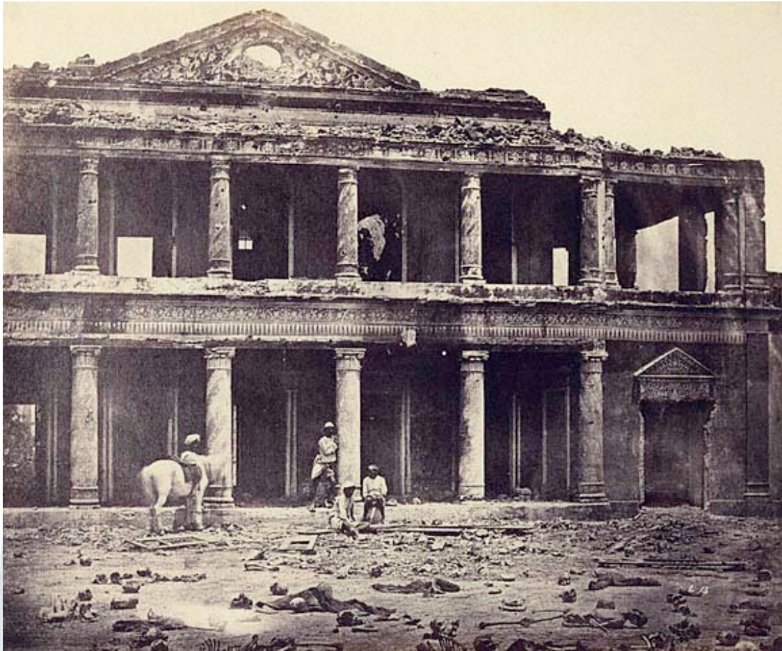
Figure 7.3.2: Interior of Sikandarabagh building
