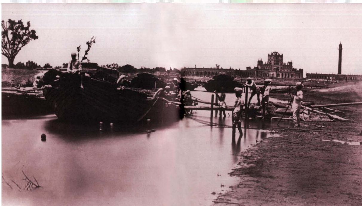
Figure 7.3.1: Bridge of boats at Delhi
